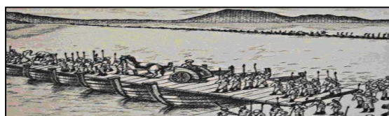
Fig. 1 Old Floating Bridge
