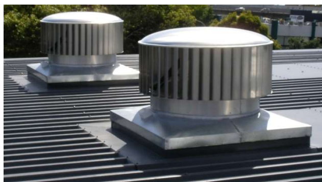
Fig 3: Rooftop Ventilator
