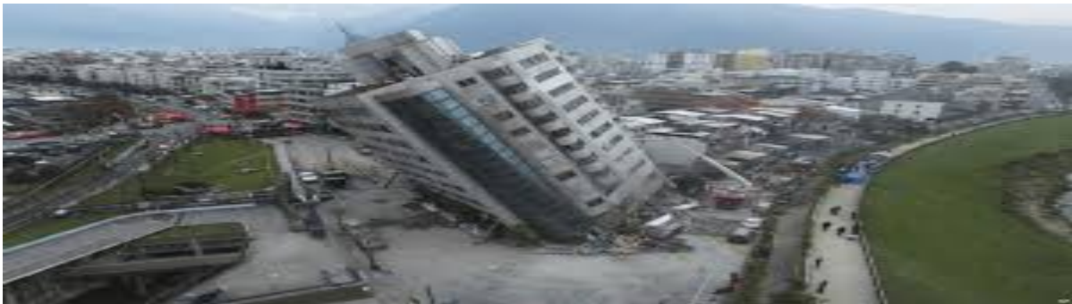
Fig.2 unequal settlement due to soil liquefaction
