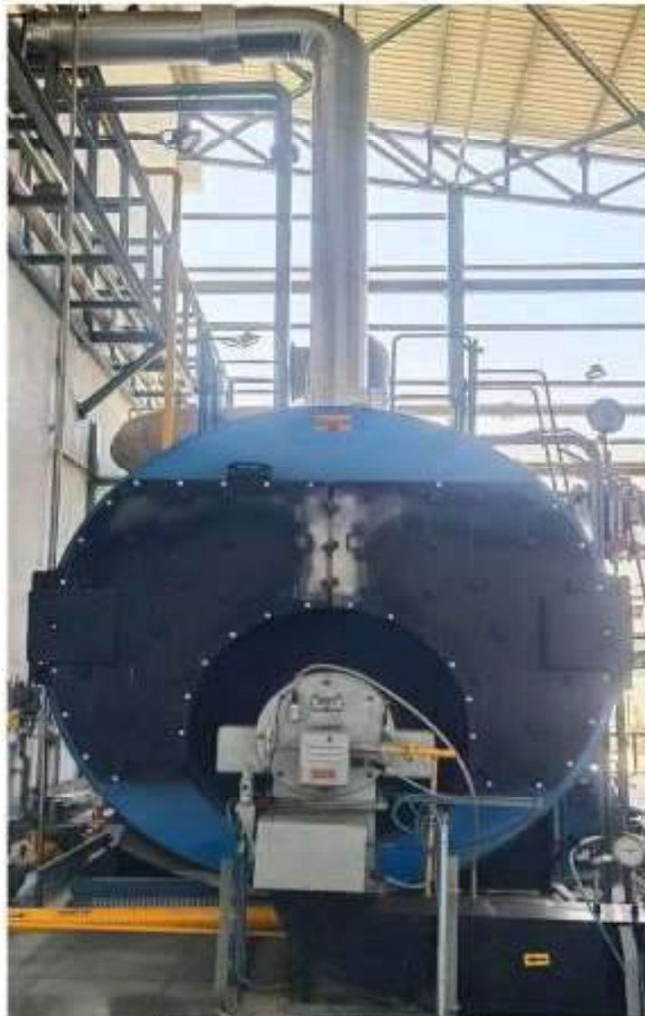
Fig 4.10 Horizontal fire-tube Boiler
