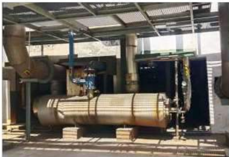
Fig 4.8 Side view of HRU
