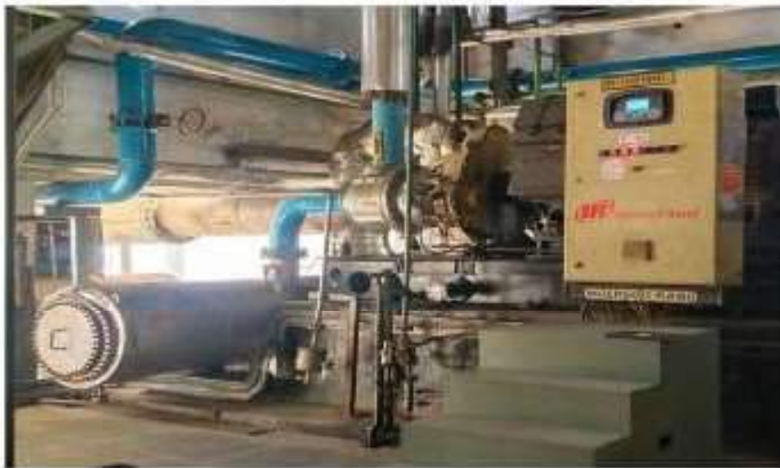
Fig 4.6 Air Compressor connected to HRU
