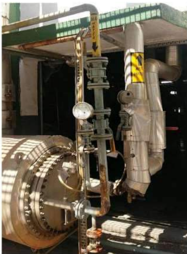
Fig 4.9 Outlet of HRU
