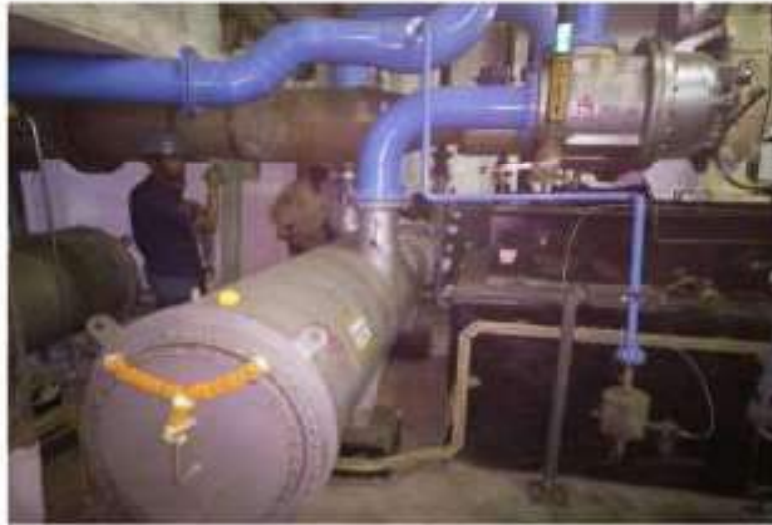
Fig 4.7 Newly installed HRU
