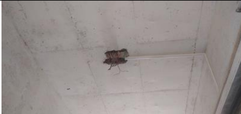
Hanging Risky Installations
