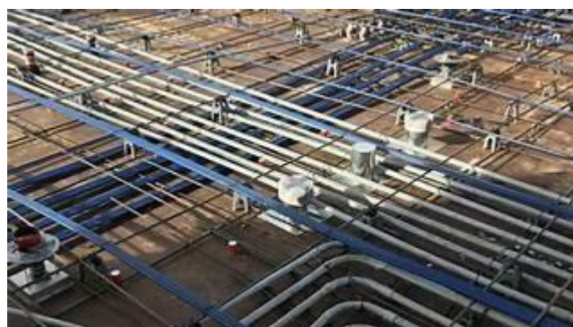
Figure 1.5 : Unbonded Post-Tensioning
