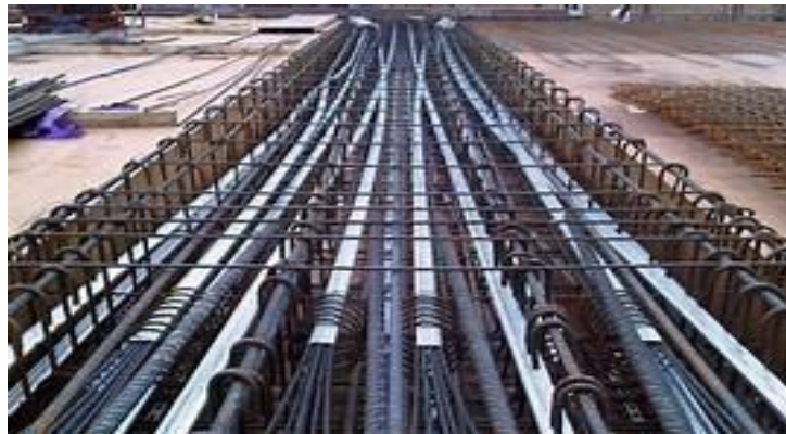
Figure 1.4 : Bonded Post-Tensioning
