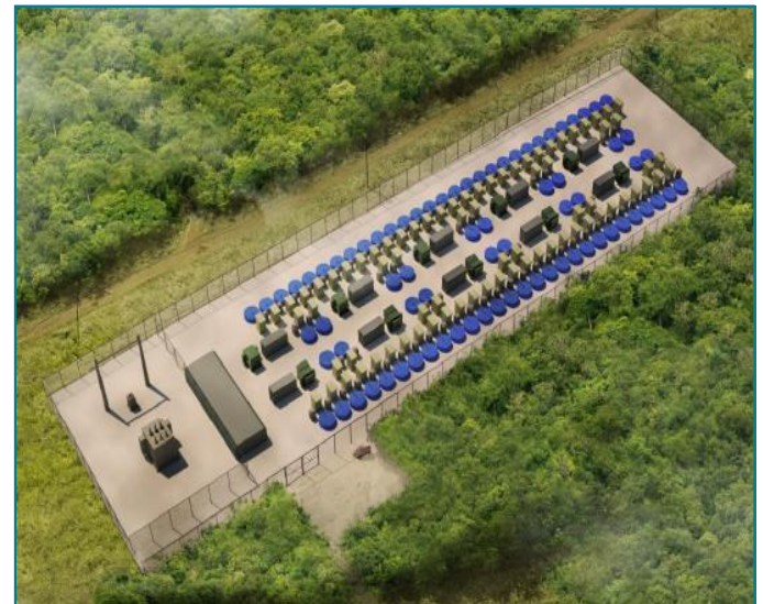
Fig.5 Representative Flywheel Energy Storage Module
