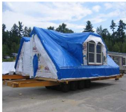
Fig. 3.1 Transportation of modules by truck
