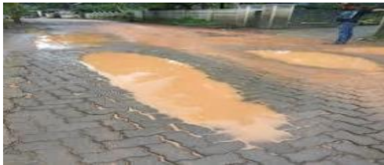
Fig - 2.2 - Water puddling on interlock pavement
