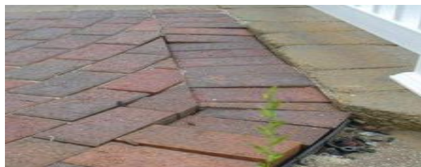
Fig-2.3- The border pavers look like they're falling off
