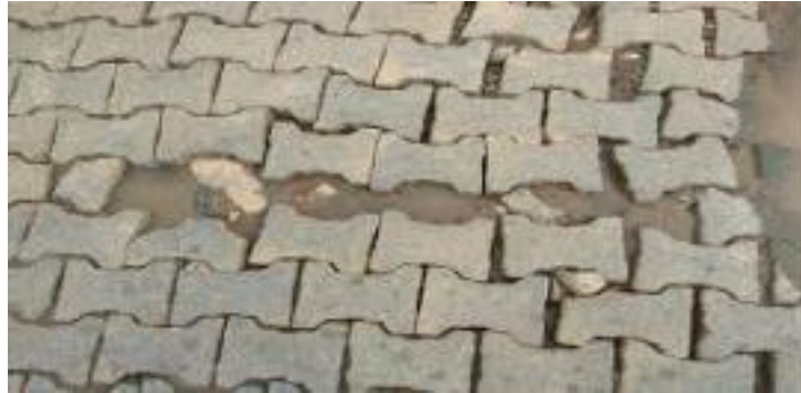
Fig -2.4- Pavers are uneven and tipping
