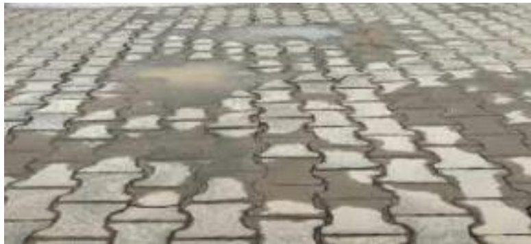
Fig - 2.1 - Paver are uneven and stay at different heights
